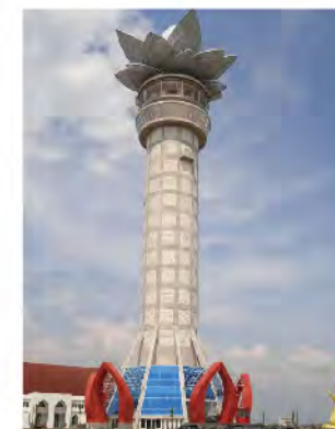
Pertamina building cilacap, Jakarta, Indonesia
