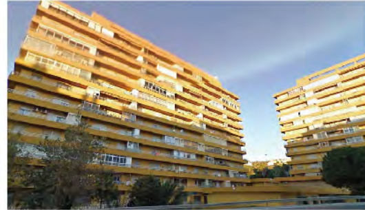
SPAIN-Staff Dormitory, Spain
